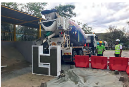
Demonstration of Agilia self-levelling concrete at the CDL of Lafarge Malaysia.
