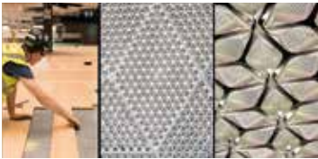
With magnetically fastened wooden flooring, sound-absorbing ceilings and integral lighting, Bloomberg headquarters in London is the most sustainable building of its kind.
