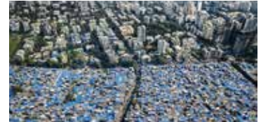
The blue in the informal settlement in the lower part of the picture is not solar modules but plastic construction elements.
