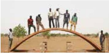
Francis Kéré used mockups as guides for illiterate construction workers.
