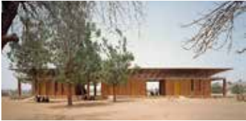
The primary school in Gando is built of clay, a material that no longer had a good reputation among the local population.
